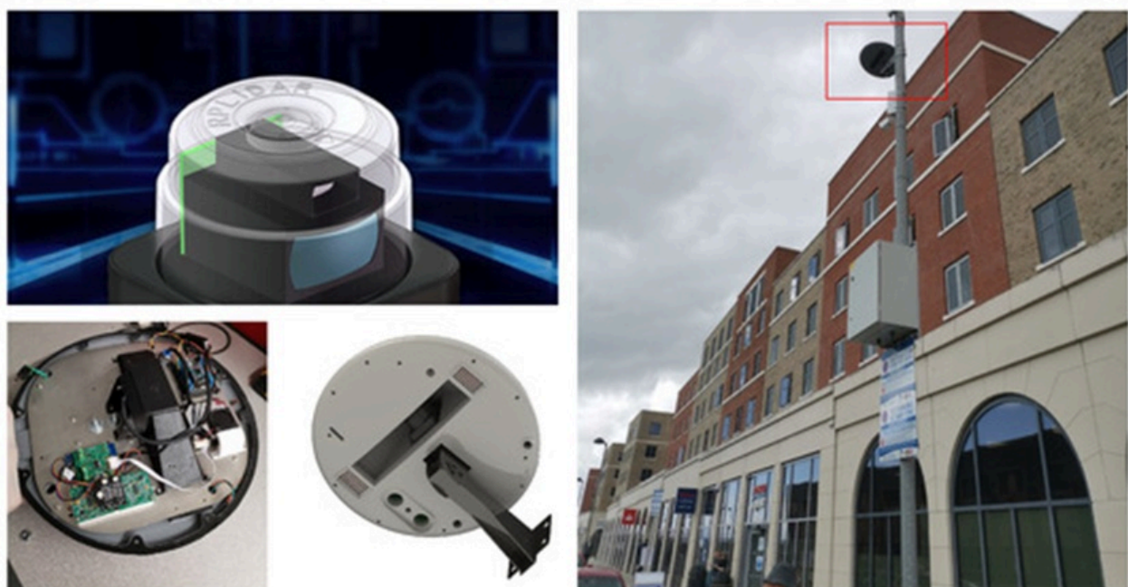
Figure 11. LiDAR hardware installation.
